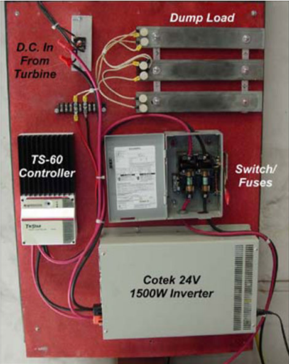
Example Illustration of Wind Turbine Wiring Components
